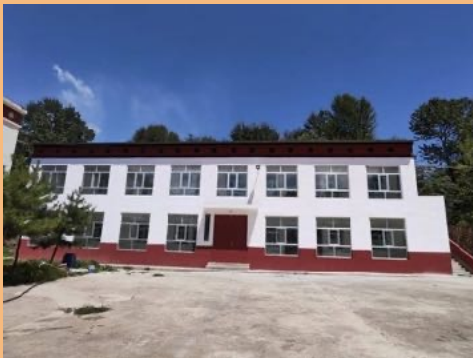
After the renovation
